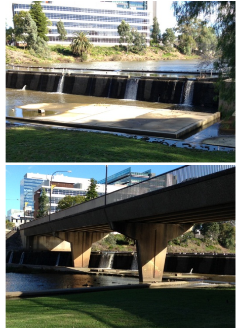
Marsden Street Weir Bernie Banton Bridge
